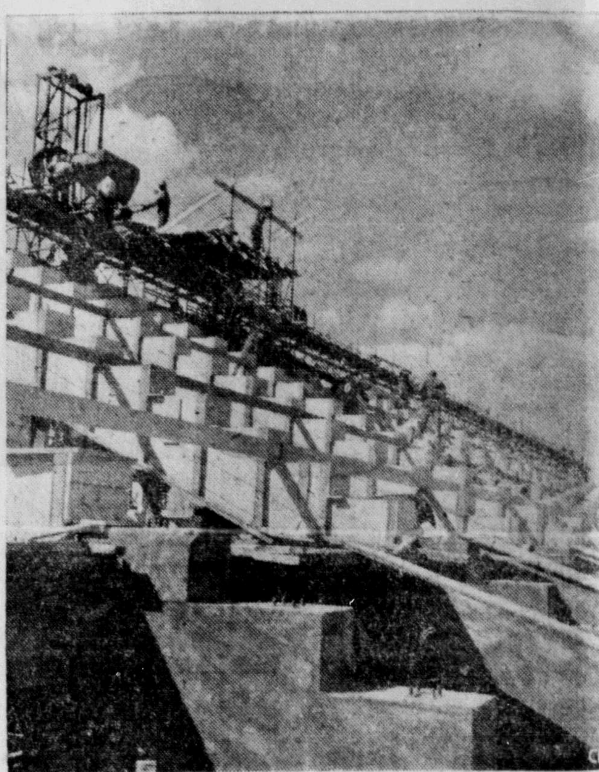
ANOTHER LOAD OF CONCRETE is poured into wooden forms for Winnipeg's $500,000 stadium. It is estimated more than 26,400,000 pounds of concrete will be used in the structure. Official opening is planned for August 14 and an exhibition football game is scheduled August 15 between Winnipeg Blue Bombers and Ottawa Rough Riders.
