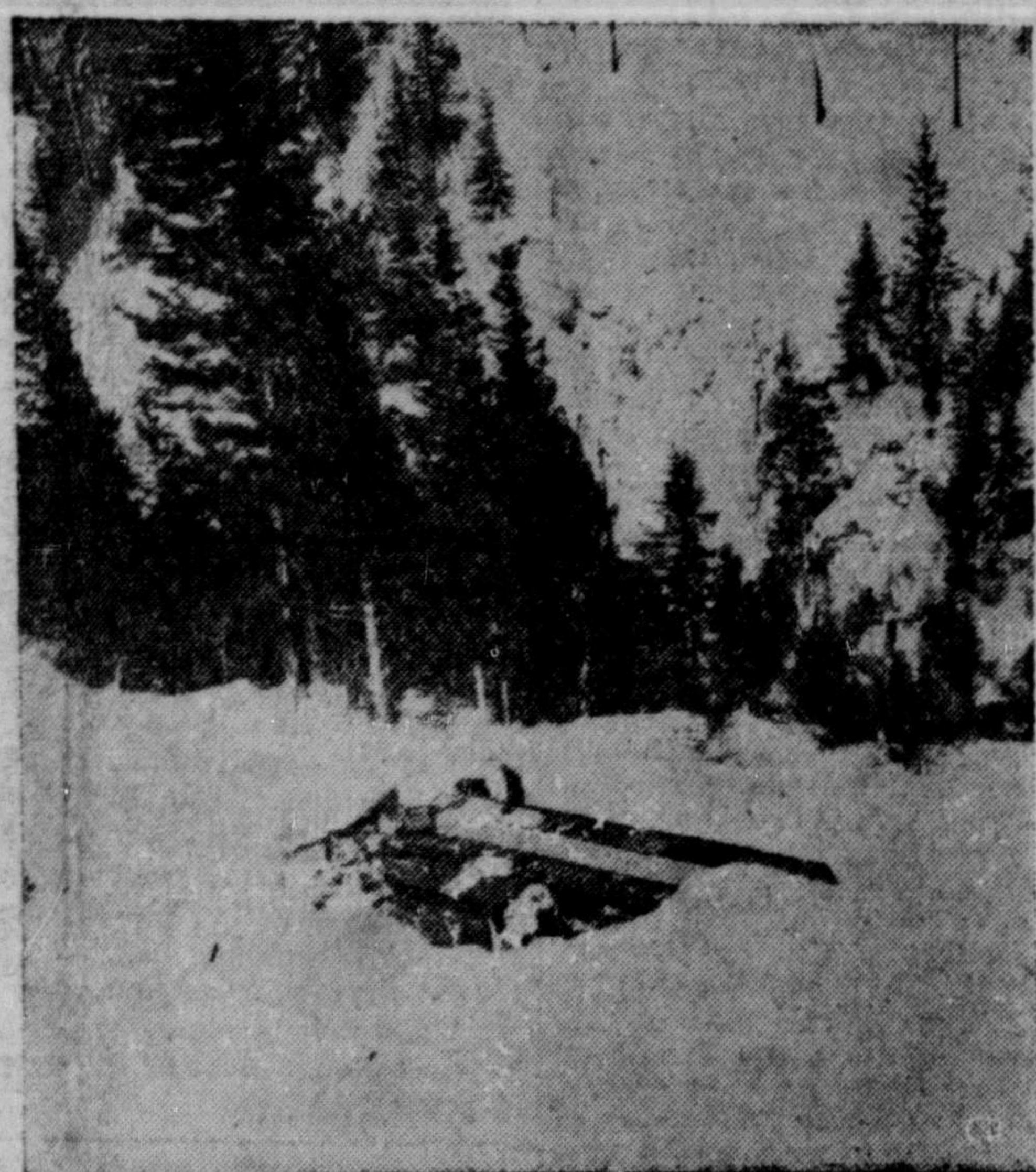
ONE OF THE BIGGEST salvage jobs in the history of B.C. railroading ended in Coquihalla Pass Saturday when this 140-ton diesel unit was put back on CPR tracks. The $240,000 unit plunged 120 feet down the mountainside Jan. 28 after it hit a snowslide at Iago, 114 miles east of Vancouver. About 50 men worked with two 100-ton cranes, anchored to the track, and a homemade 'ladder' winching machine on a flatcar to retrieve the diesel. It had to be moved 175 feet along the slope before it could be inched upwards over skidways placed atop rock outcroppings. The unit is being towed to Calgary for repairs.
