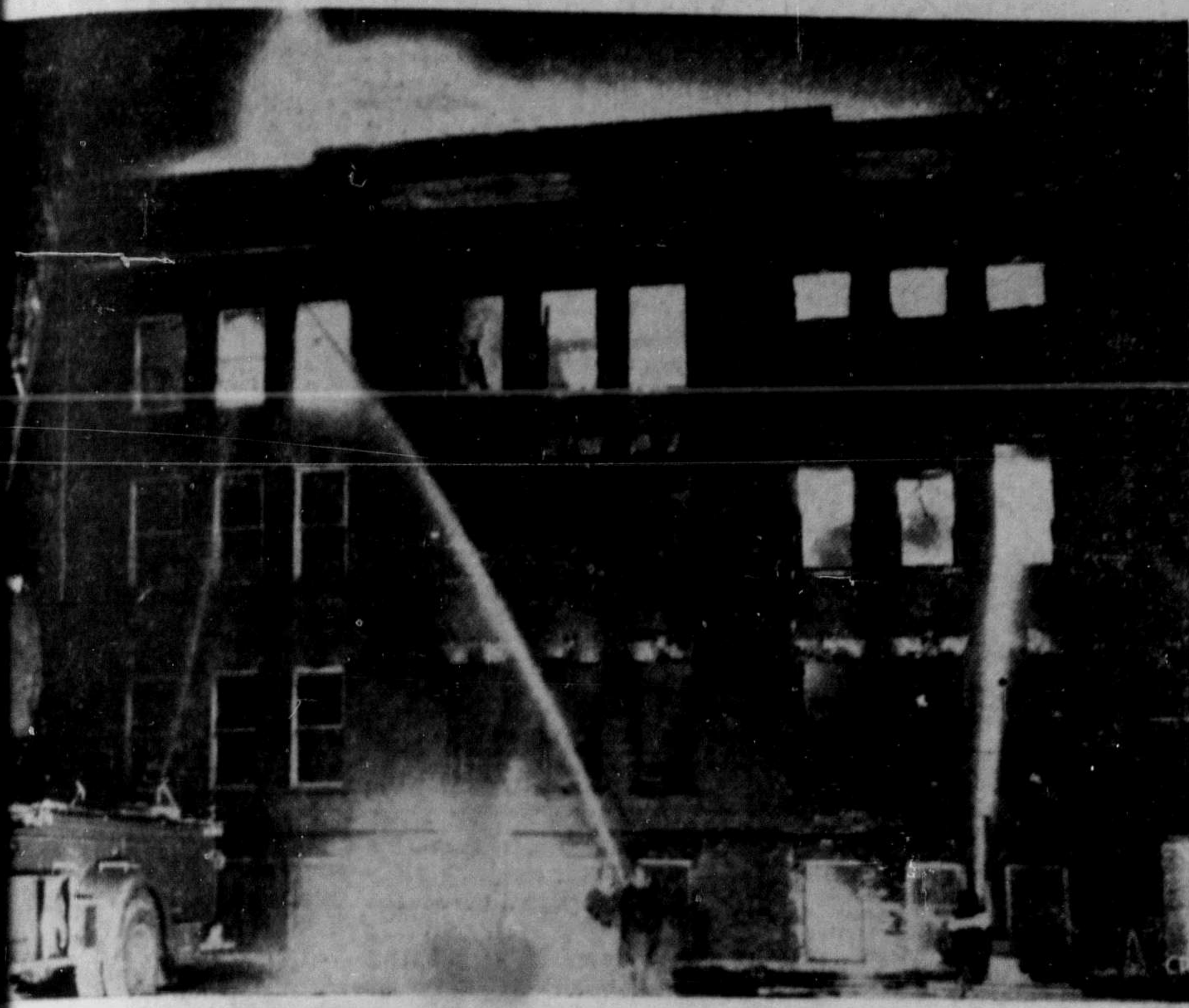
Fire Destroys School
