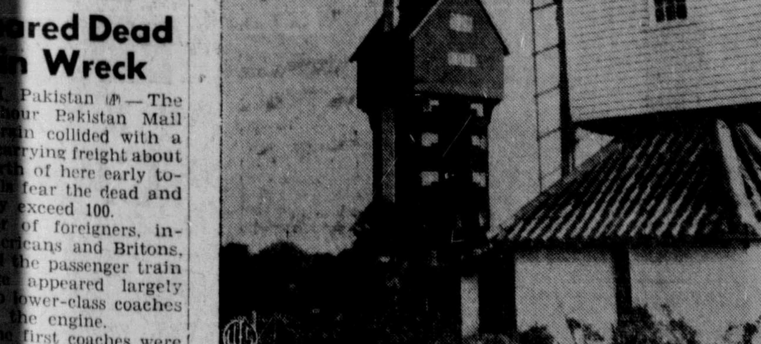
THOUGH THERE'S a hint of Holland in the windmill appearing in the foreground, the tall house is a landmark on the British countryside at Thorpe, Suffolk. Actually it is a water tower which supplies a nearby village. Four floors of living quarters have been built beneath the tank, and skillful painting has completed the illusion of "a house in the clouds"
