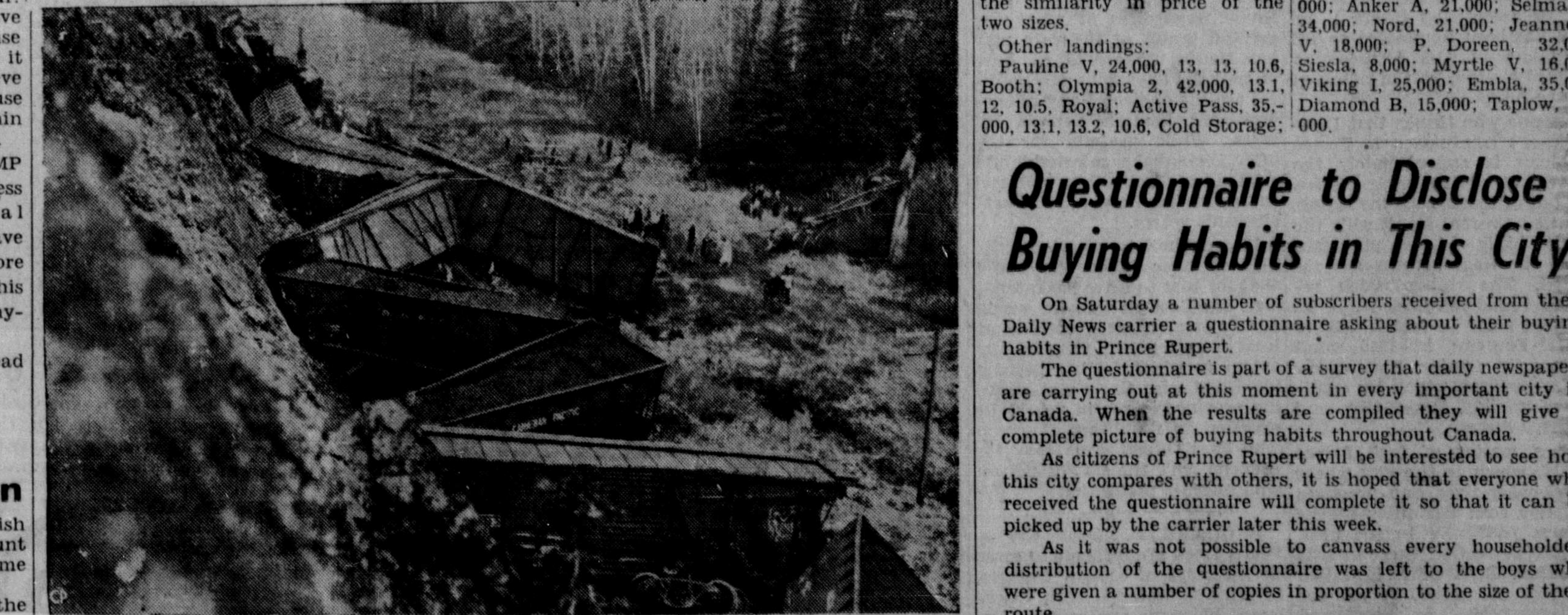
Ten crumpled freight and coal cars piled up when a 42-car train was derailed in the Crows Nest Pass, east of Blairmore, Alta. The derailment caused extensive damage to the rails but no one was injured.
