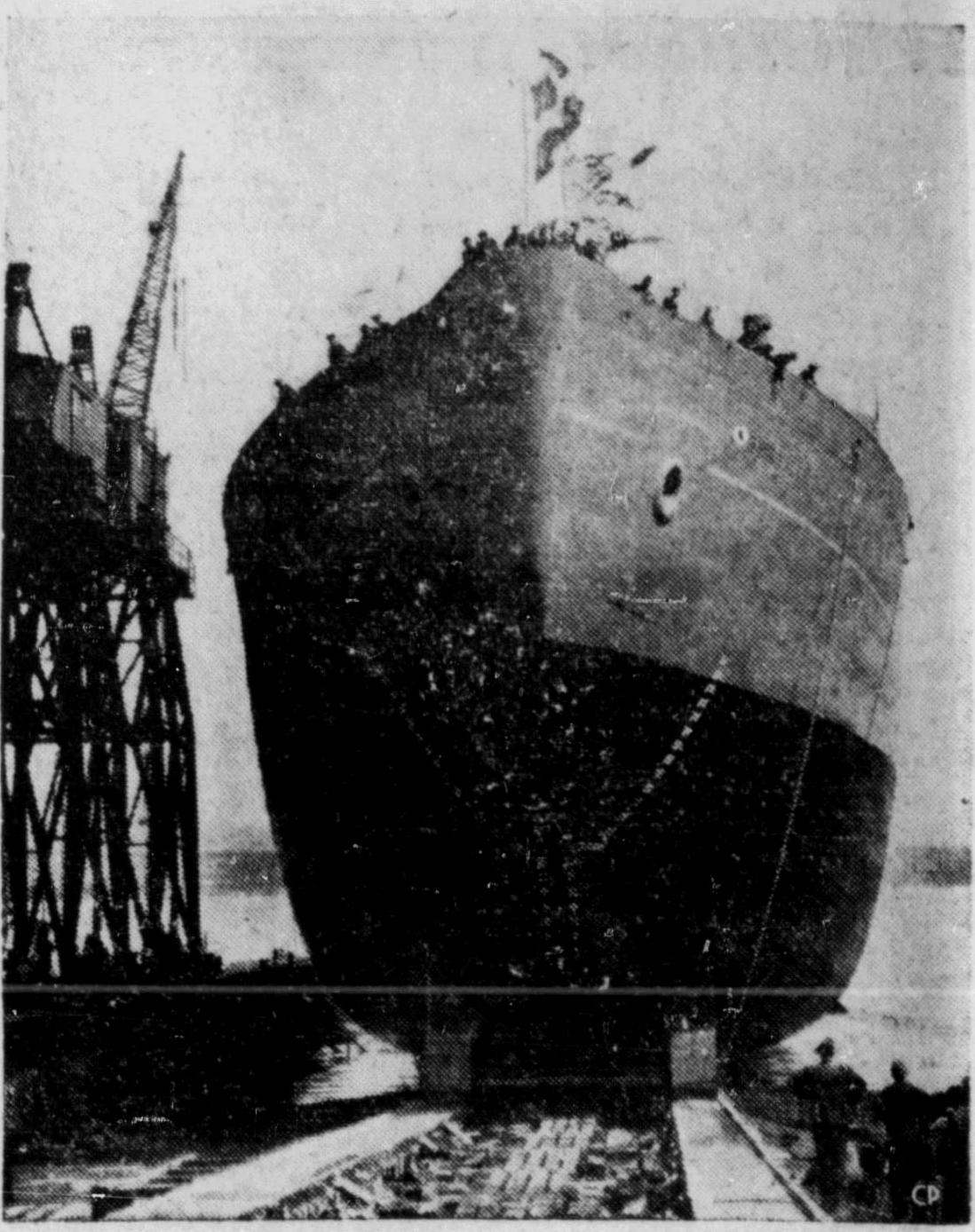
LARGEST ICE-BREAKER—The 3,100-ton hull of the d'Iberville. the continent's largest ice-breaker, slips into the St. Lawrence river at Lauzon, Que., where it was built. The Transport Department's new ship is able to cruise 12,000 miles without refueling and is expected to reach Arctic regions where no previous Canadian ships have touched. The d'Iberville will be equipped with two helicopters for photography and scouting. (CP PHOTO)
