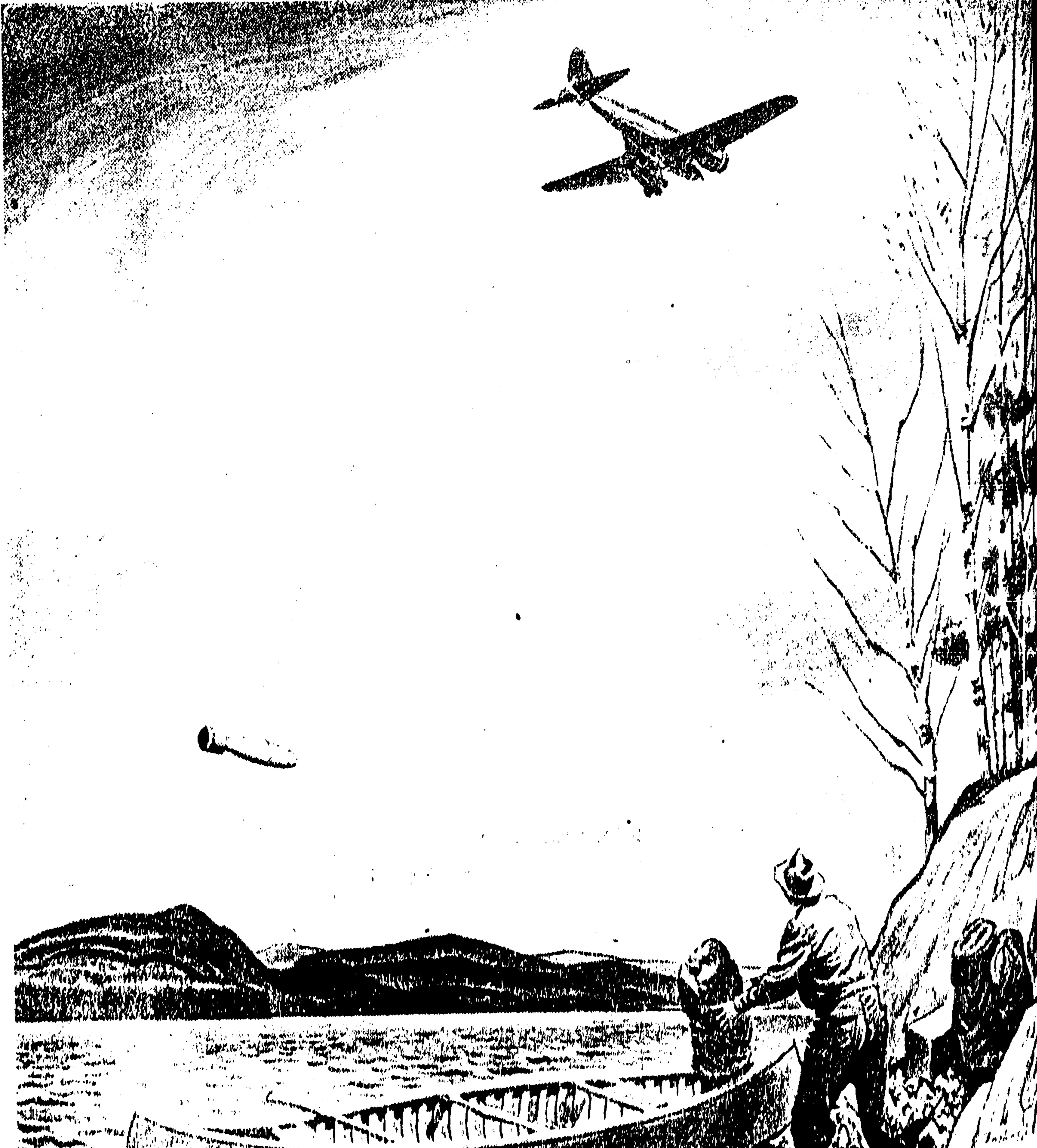
Towing highly sensitive instruments from an aeroplane, Inco's air prospectors have been able to locate promising mineral deposits hidden beneath the earth's surface. Then by referring to a continuous strip of photographs taken from the plane, they can point likely areas to be worked by ground prospectors.
