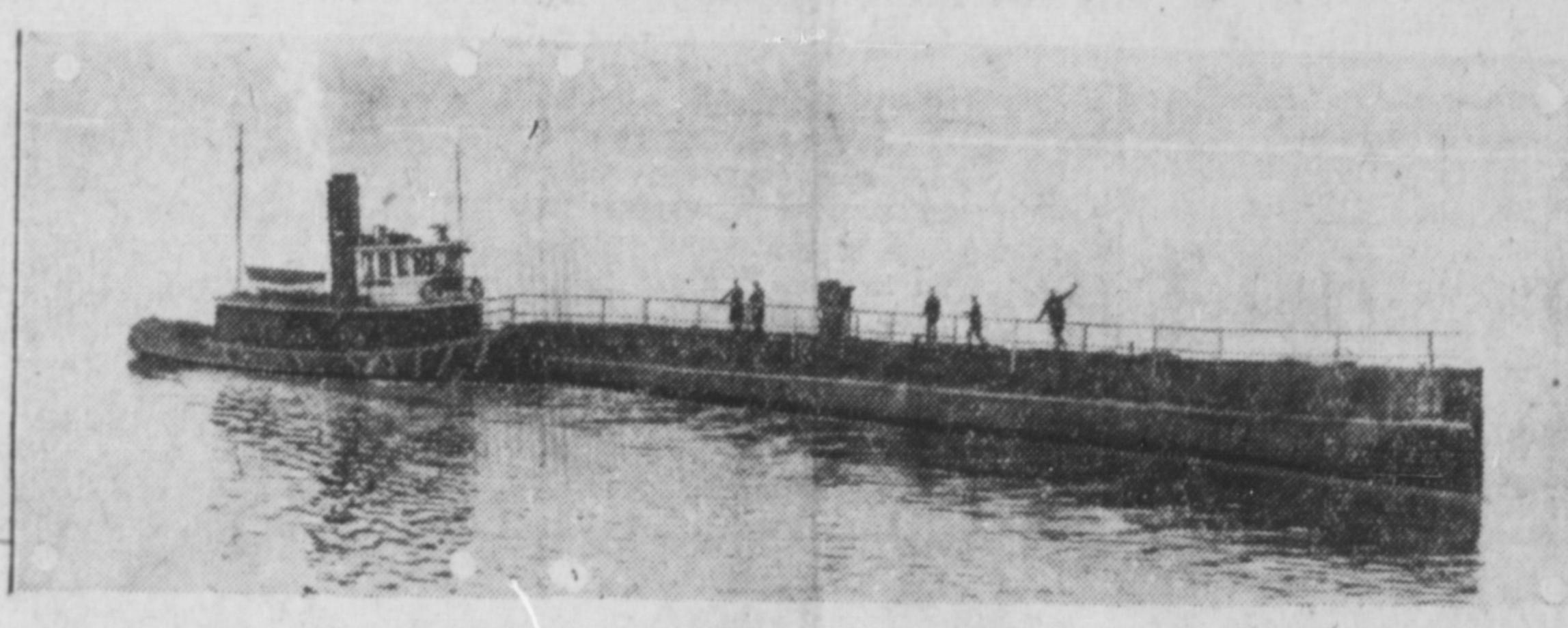
After extensive overhauling at Philadelphia, Nautilus, once navy submarine O-12, proceeds to Camden, New Jersey, to be equipped with telescopic ice drills to be used by Sir George Hubert Wilkins' expedition to North Pole.
